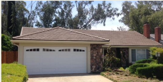
Last house to replace cedar shake roof
