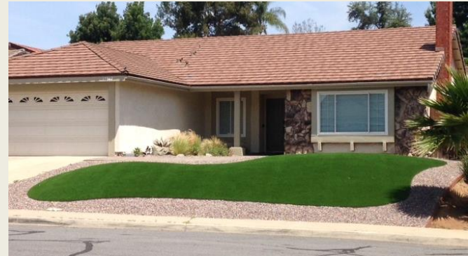
Artificial turf works even on steep slopes
