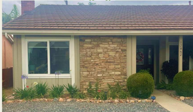
Decorative stone replacing brick
